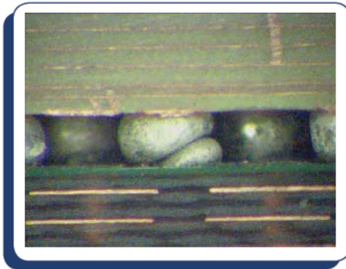
Figure 3-2: A head-on-pillow defect that was verified optically without the aid of mounting and polishing.
